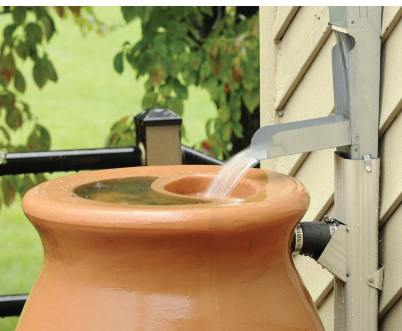
When it rains, it pours! Your roof is likely the largest contributor of runoff on your property. Say you have a 10-metre by 12-metre roof surface. During a single 2.5-centimetre rain event, 3000 litres of rainwater can run off your roof. Multiply that over the course of the year, and that's a lot of water just washing away.
