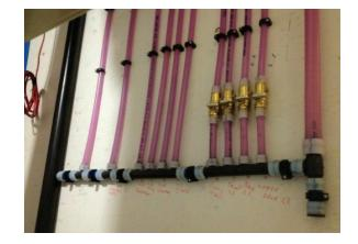
**TOP LEFT:** Modular cisterns are available for different surface-weight loadings. To be used as a cistern, they are wrapped in a waterproof membrane, using the same technology and installers as are used for basement radon-proofing. **TOP RIGHT:** Cartridge filter canisters below (blue) and UV disinfection above. **BOTTOM:** Purple-pipe distribution manifold in a home with rainwater used for toilet flushing.
