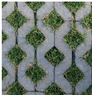
LEFT: Grasscrete in-situ forming system, courtesy Eagle Lake Landscape Supply.
