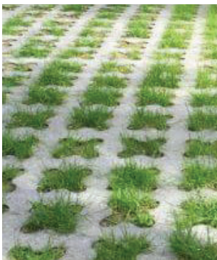
LEFT: Grasscrete in-situ forming system, courtesy Eagle Lake Landscape Supply.
