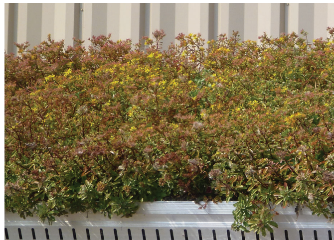
TOP: Mixed native extensive green roof irrigated from a cistern that harvests parking lot runoff.
