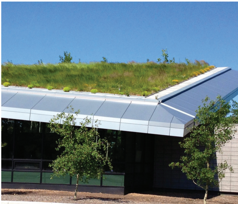
ABOVE:| Innisfail Library
